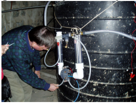
Water purifier being installed
