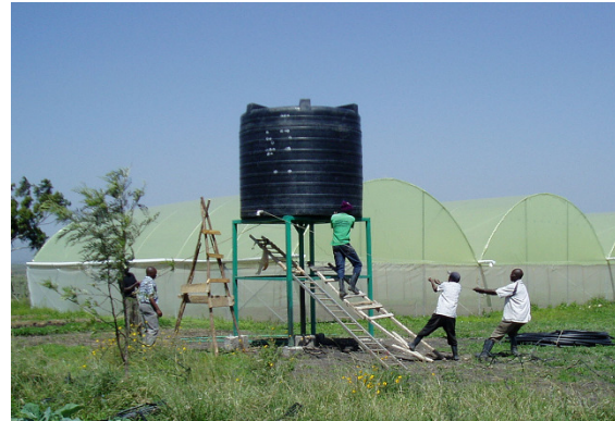
Overhead Greenhouse irrigation tank
