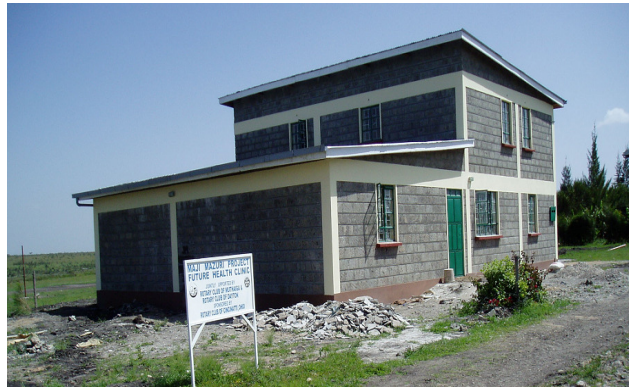
Newly completed clinic building
